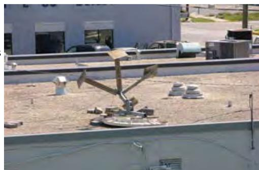
*This satellite dish simply sat on the roof ballasted with concrete pavers. Wind-blown dishes can tear roof membranes.*
