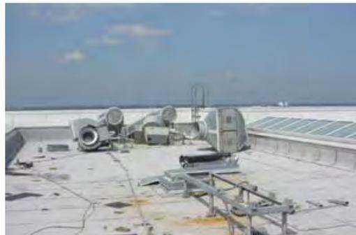
*These fans were on vibration isolators that did not provide uplift resistance. The fans blew away because the wind pressure exceeded the weight of the fans.*
