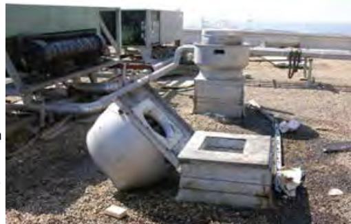
*This fan was not adequately attached to the curb. Fan attachment easily can be evaluated and inexpensively upgraded if needed, thereby avoiding a substantial amount of water infiltration.*
